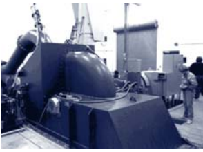
Water turbine like those installed at Beochlich
