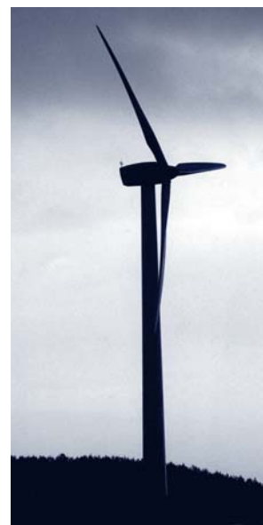
Part of the wind cluster at Haverigg II
